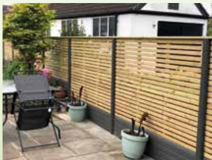
ex50mm x 18mm used for fencing panels
